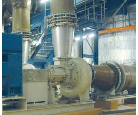
FGD pump, used in flue gas desulfurization in a power plant
