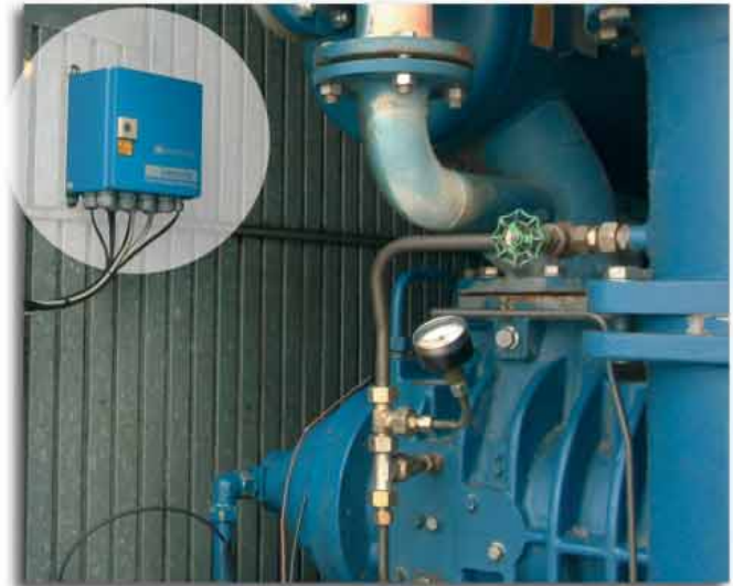
Monitoring with the VIBNODE® online monitoring system
